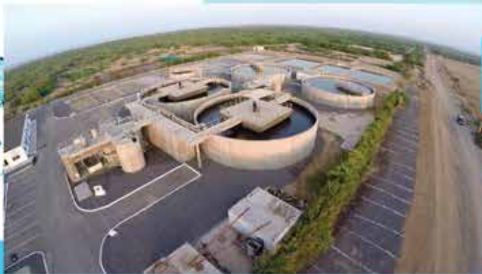
View by drone of the treatment plant
