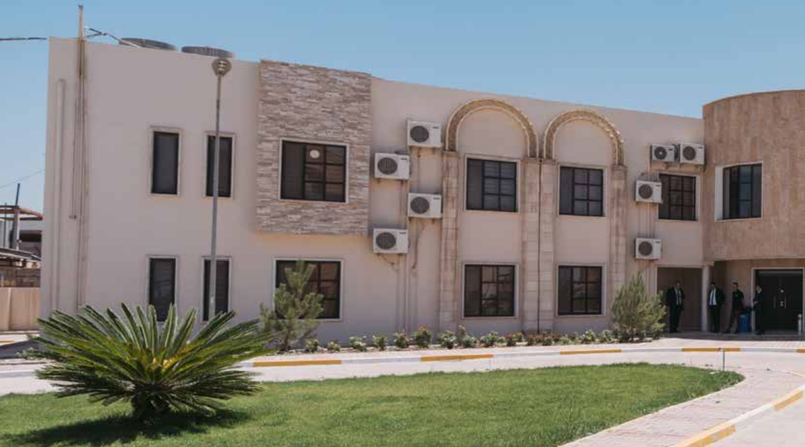
Central training center of the Ministry of Electricity (KRG) © Luthardt GmbH
